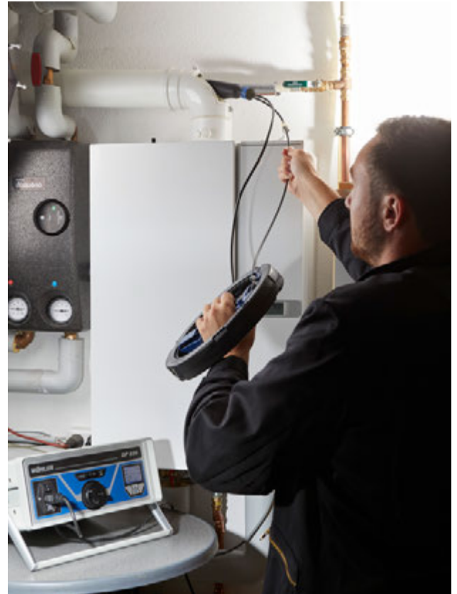
Tightness testing of all flue gas systems.
